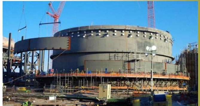
In February 2016, all six sections of the third course of shield building panels were set in the V.C. Summer Unit 2 Nuclear Island. Weighing approximately 30,000 pounds and spanning 40 feet long, each panel is welded together, and then concrete is poured inside the panels to create the shield building. When complete, this reinforced concrete structure will surround the containment vessel for another layer of safety.
